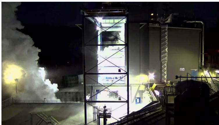
Fig. 16: Test Facility P5.2 during hot-run with ULPM/Vinci® engine
