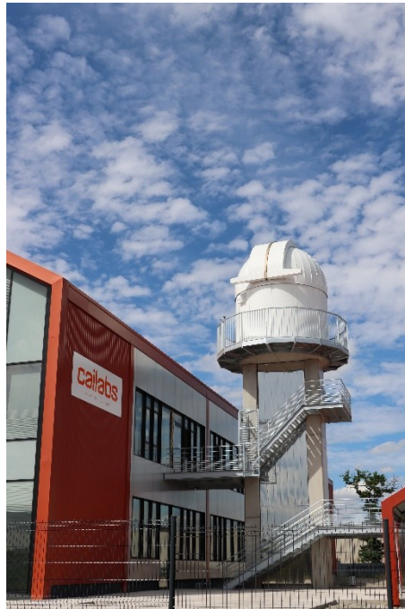
Figure 1 – Picture of the OGS on its concrete tower.
