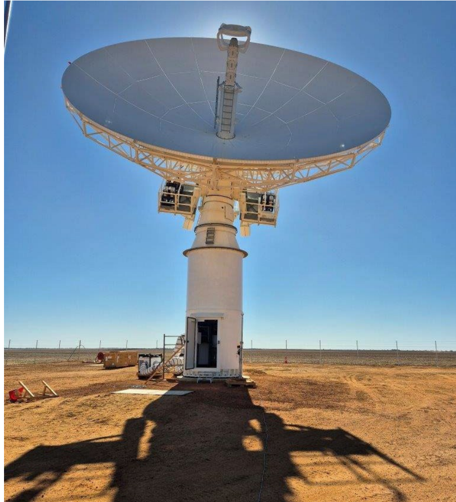
Figure 4-1 Construction of new 13.5-m class antenna in Western Australia aimed for Lunar support with X/S TT&C.
